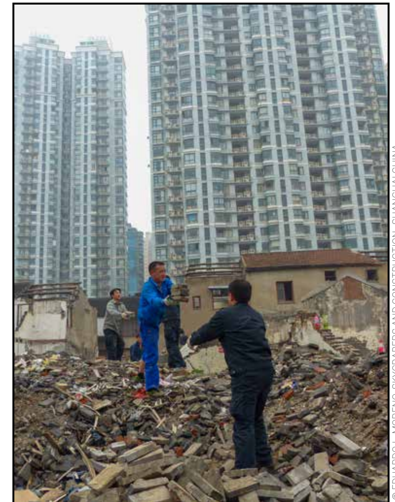
© EDUARDO L. MORENO. SKYSCRAPERS AND CONSTRUCTION, SHANGHAI, CHINA
